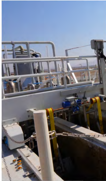
Grit & Grease Scraper Bridges
