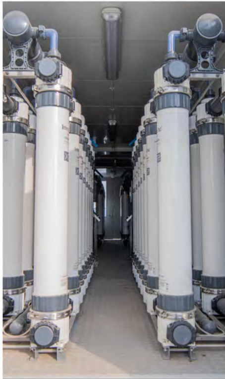
Containerized Ultrafiltration
