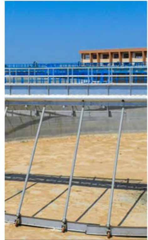
Rotating Scraper Bridges
